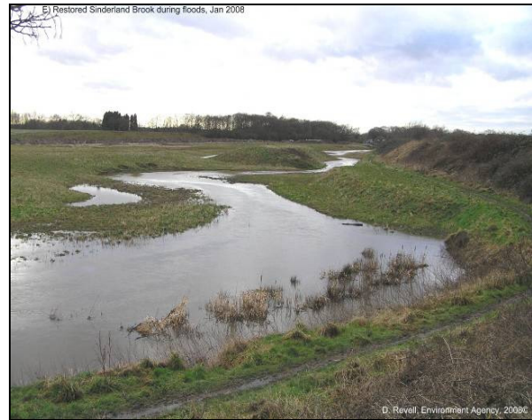
Sinderland Brook after the flood alleviation works, showing the meandering channel re-connected to its floodplain
