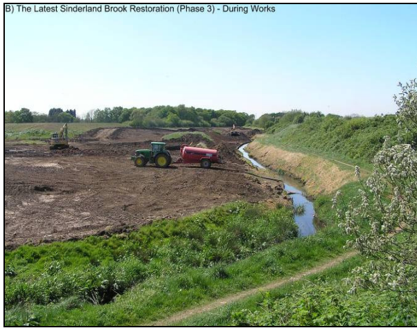
Sinderland Brook during works (photo courtesy of Environment Agency)
