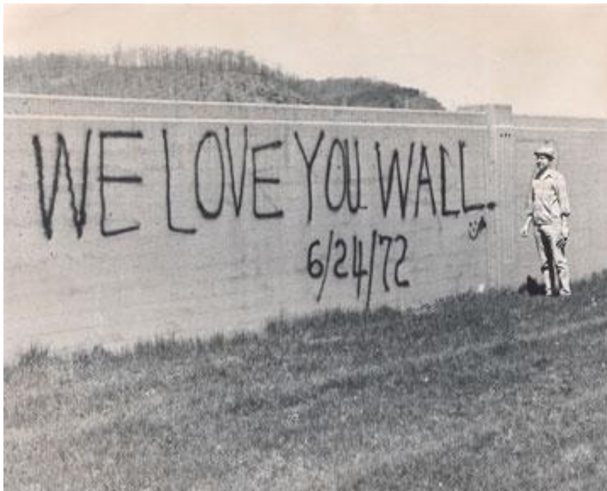
Hurricane Agnes' floodwaters were within inches of overtopping Sunbury's flood wall (Photo courtesy SRBC archives)
